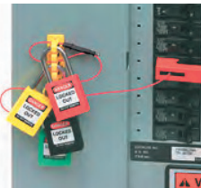
4. For group lockouts, run key through multiple loops in lock rail and apply locks. No hasps required! (Not recommended for use with multilock hasps)
